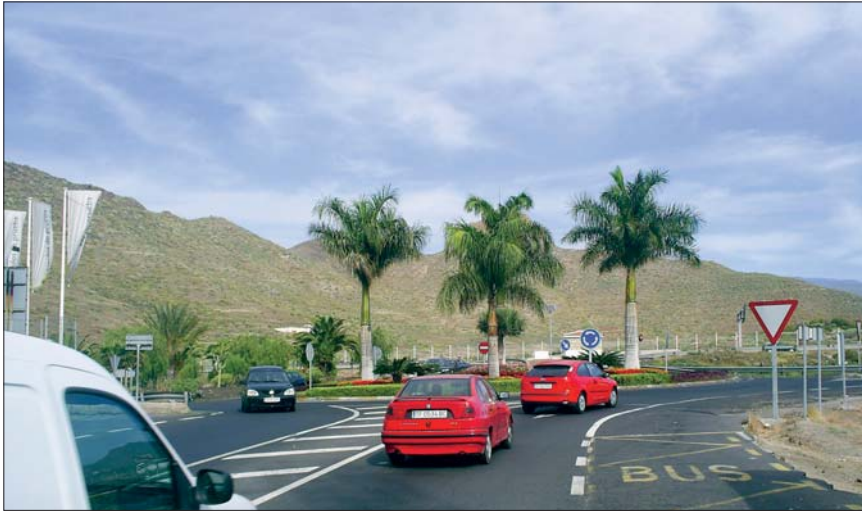
Much more work needs to be done to improve the roads throughout the Arona borough
